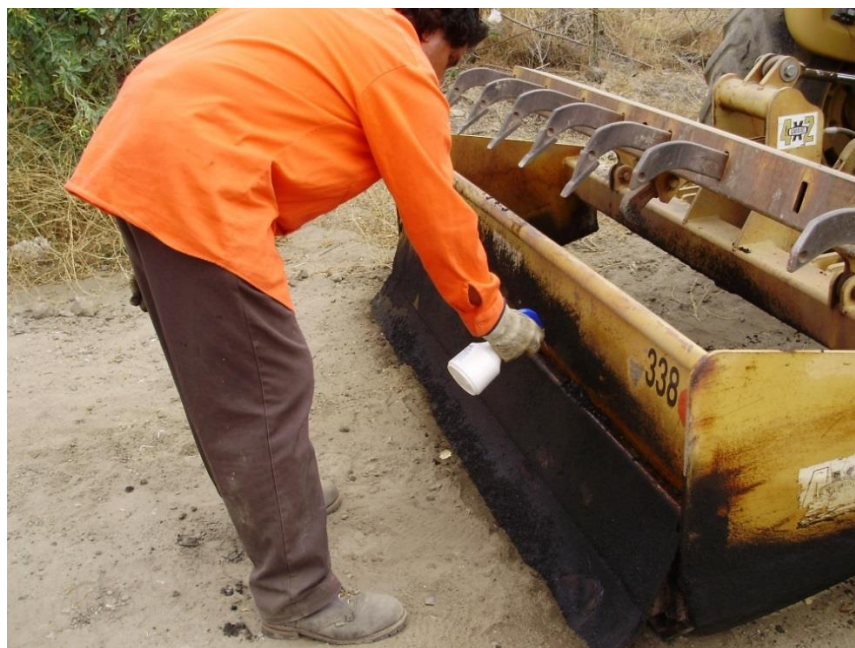
Figure 2-22 Spraying Release Agent on Tractor Scoop
