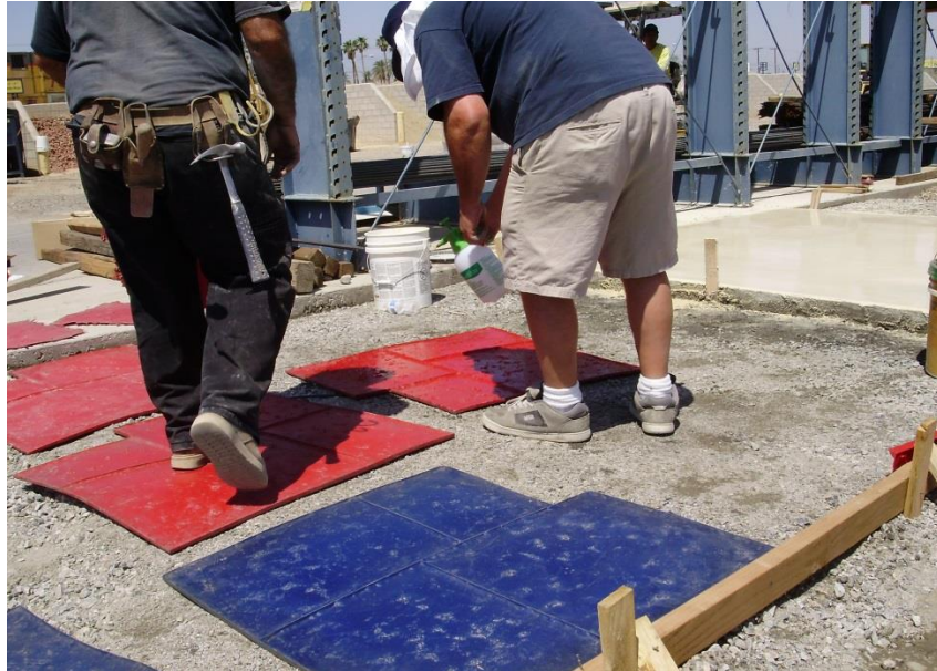
Figure 2-2 Spraying Stamp Mat with Release Agent
