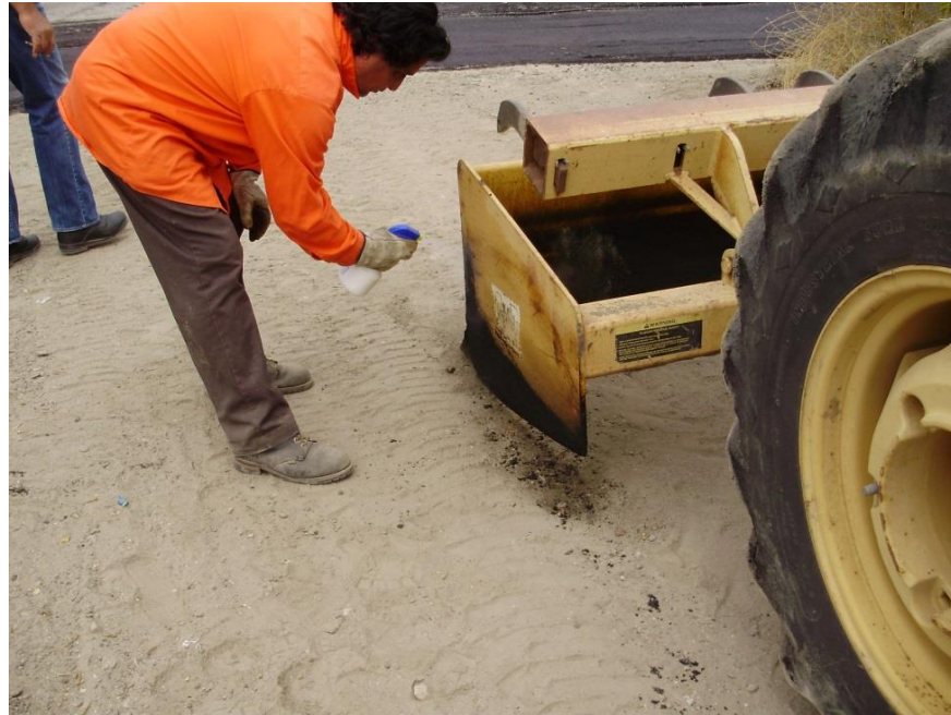
Figure 2-21 Spraying Release Agent on Tractor
